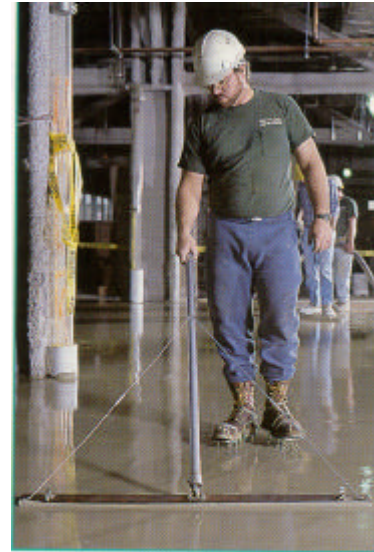
Rapid Floor Ultra always pours a smooth, level floor practically from the instant it's pumped onto the old surface or new concrete subfloor. Only minimal finishing is required.
